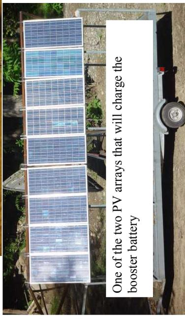
One of the two PV arrays that will charge the booster battery
